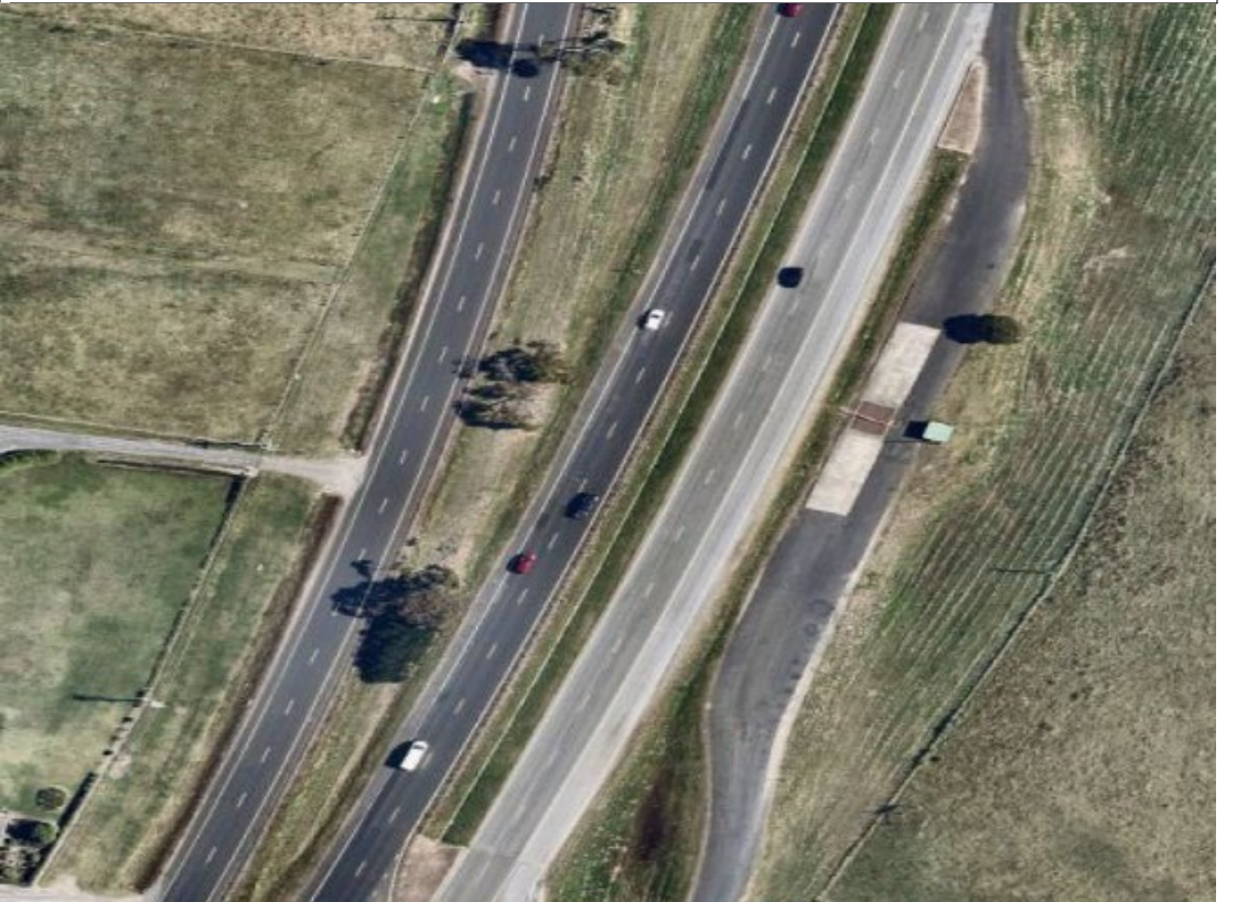
Bass Hwy / Maskells Rd / & weighbridge site, East Ulverstone
