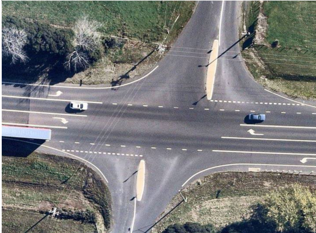
Simple 4-way Intersection – Bass Hwy / Reservoir Dr, Wynyard
