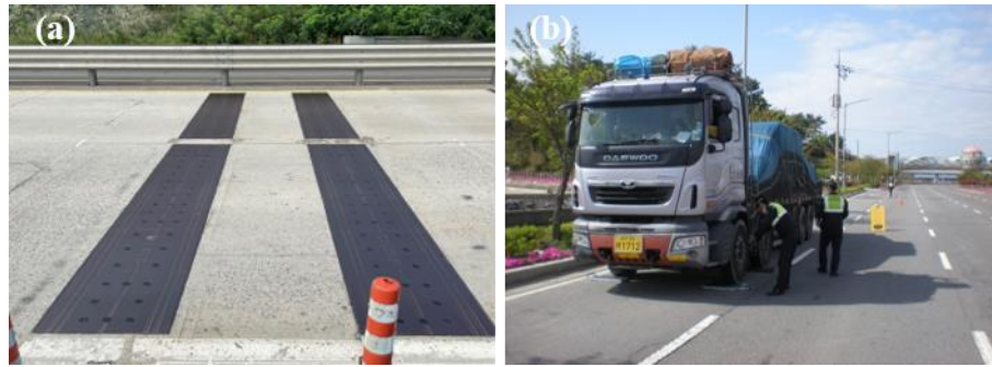
Figure 1 – (a) load cell-type HS-WIM and (b) mobile enforcement team in Korea
