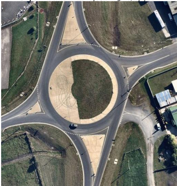
Roundabout - Bass Hwy / Calder Rd / York St, Wynyard
