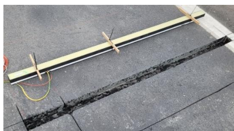
Figure 8 - Sensor installation
