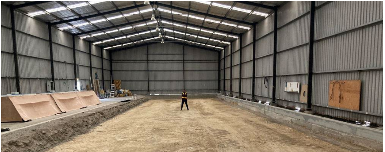
Figure 3 The test pavement subgrade and surrounding concrete walls
