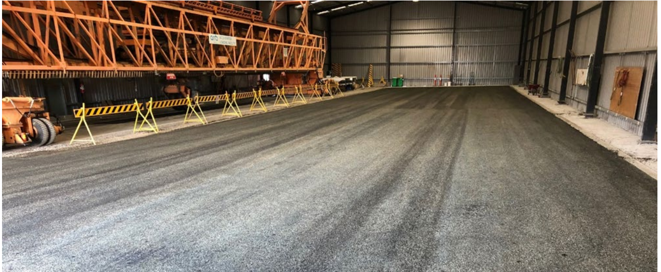
Figure 4 The test pavement after the spray seal was applied
