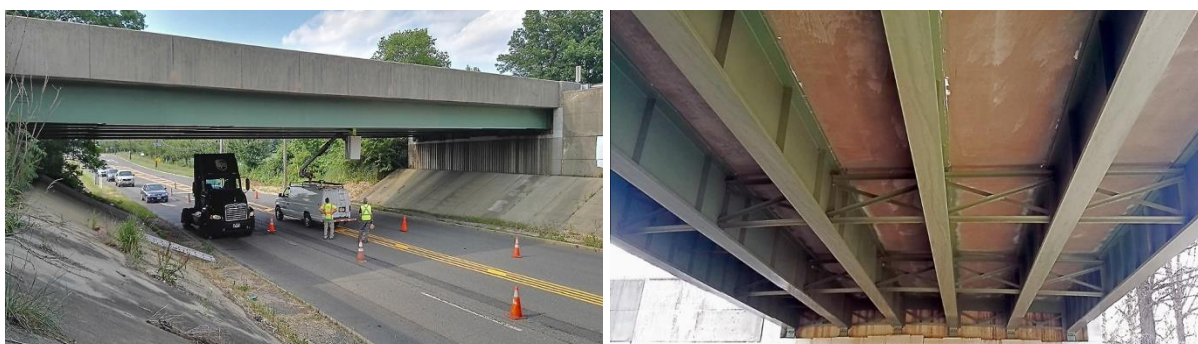
Figure 3 – Side view and view from below of Bridge B
