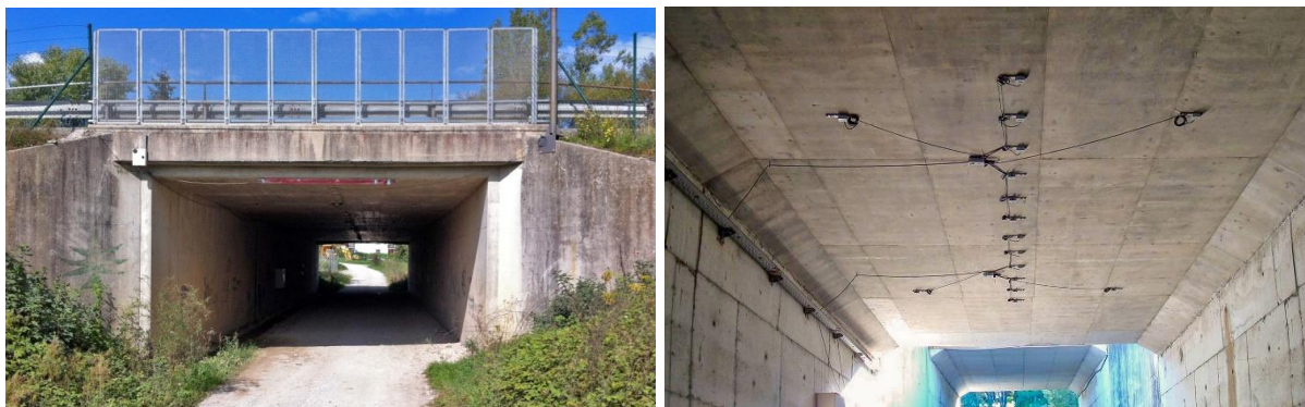
Figure 2 – Side view and view from below of Bridge A
